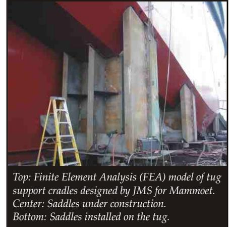
Top: Finite Element Analysis (FEA) model of tug support cradles designed by JMS for Mammoet. Center: Saddles under construction. Bottom: Saddles installed on the tug.
